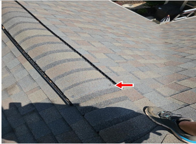
Item 5 - Item 1 (Picture)
